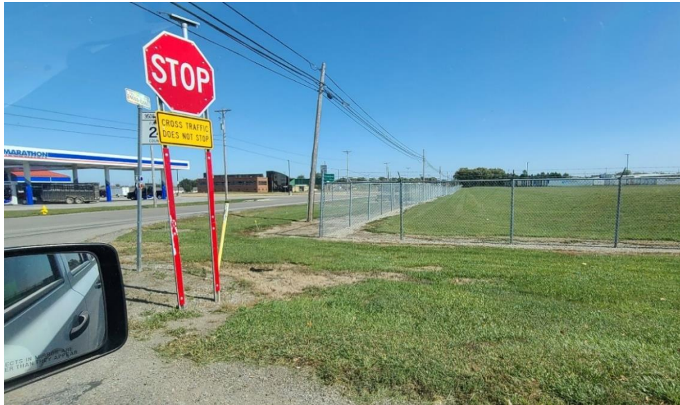
Figure 5 Northbound looking east at the stop sign
